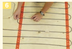
Install Therma Cable .
