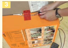
Test the integrity of the cable. Carefully read the installation guide prior to installing the heating cable.
