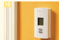
Before turning on the Therma Cable floor heating system, make sure all construction materials are well cured (check manufacturer instructions).
