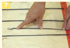
Install floor temperature sensor.
