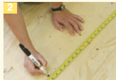
Clean the subfloor and mark the work site.
